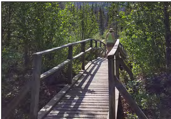
A bridge traversing a ravine that can fill up with snow melt or heavy rains, on the Rock Glacier Trail in Kluane National Park and Reserve, Yukon, Canada. Photo: Dan Dyck.
