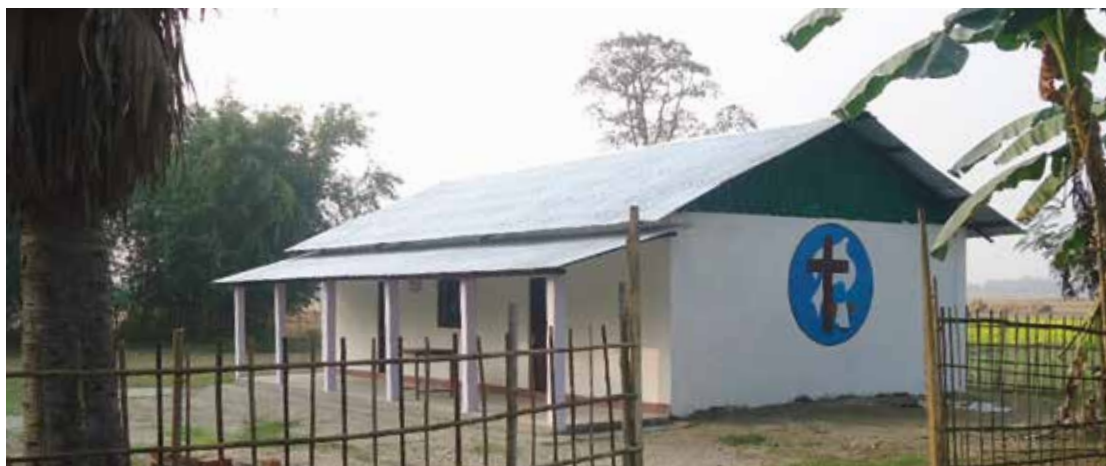
The new concrete church building in Babiya, Nepal, constructed with assistance from MWC Global Church Sharing Fund.
