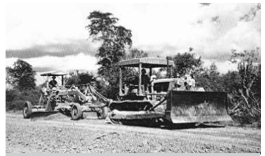
Grading the Transchaco Highway
