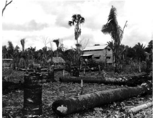
Clearing land in Belize
